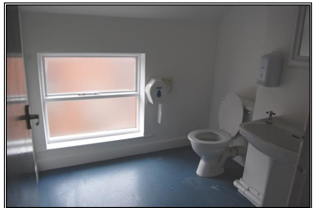
Second Floor WC
