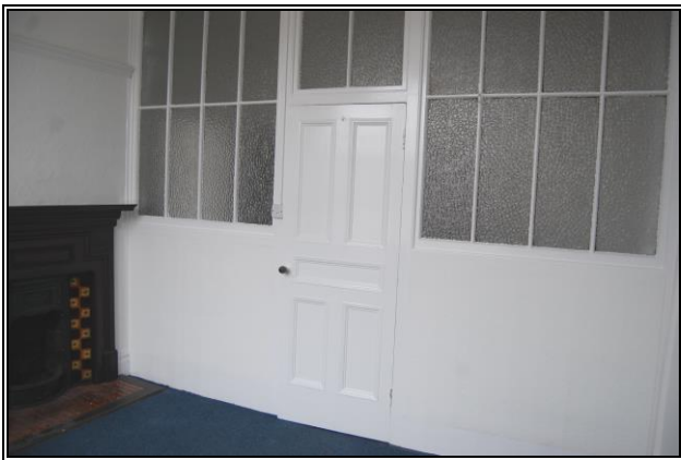
First Floor Office 2
